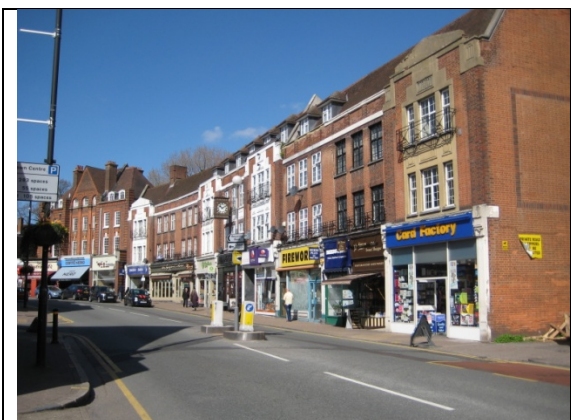
High Street with no 134 in the foreground.
